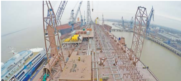
| Conversion Works at China Yard
