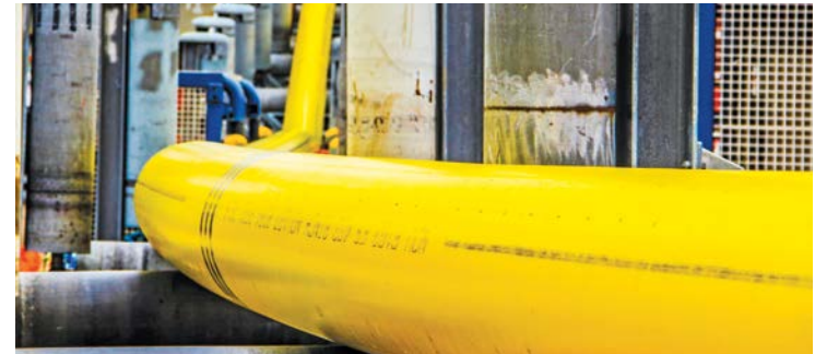
| Transpoiling of flexible flowlines
